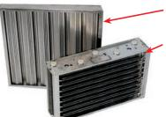
The **BAFFLE FILTER** & the **EAC CELL** must be cleaned daily.
