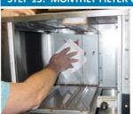
EVERY 30 DAYS, remove all 3 filters. Use an approved cleaning solution, or the Foaming Crystal Cleaner & a clean sanitized towel to thoroughly clean the inside of the hood plenum. USE CLEANER SPARINGLY WHEN ATTEMPTING TO CLEANING FAN BLADES.
