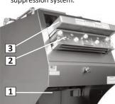
[1] Stainless steel Baffle Filter removes a portion of the grease from cooking vapors.
